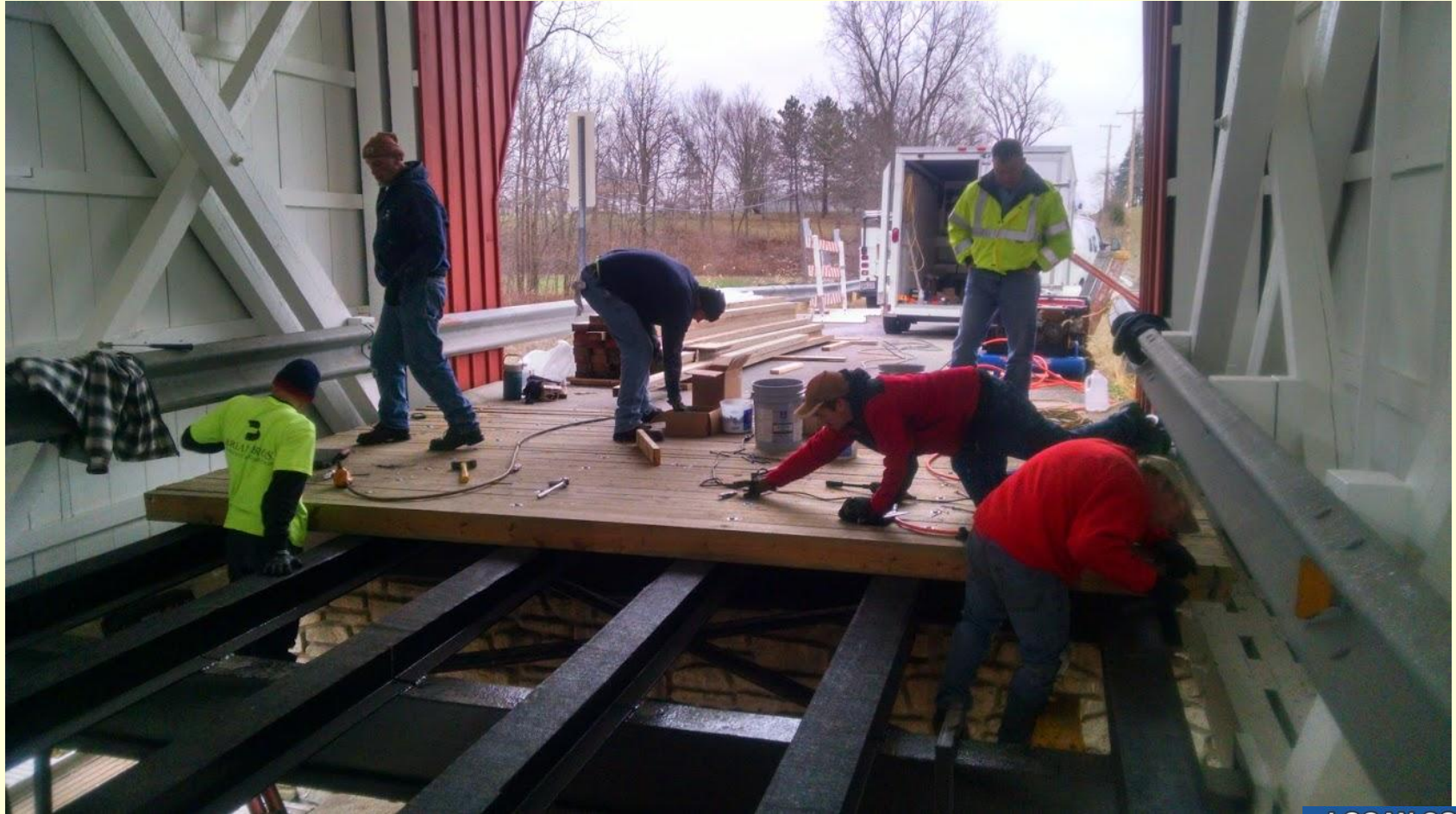
Installing the new timber deck
